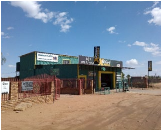
Figure 18: A commercial property situated along the arterial road. Source: Charman personal collection, 2023
